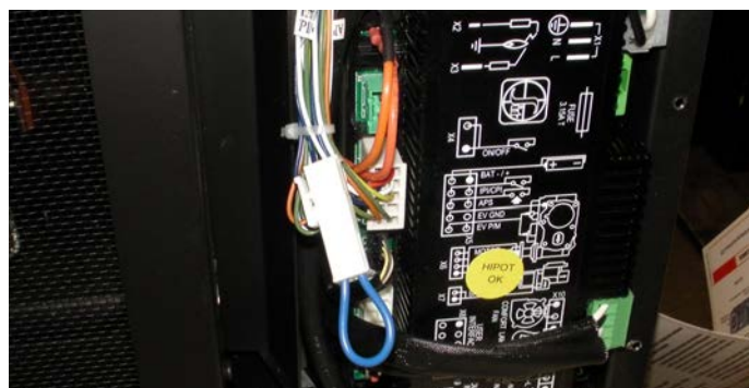
Figure 19.c Raccordez le câble de raccordement
