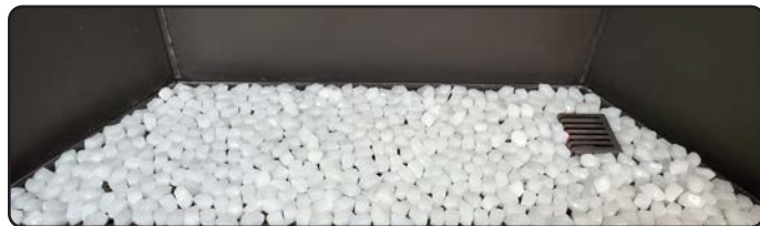
Figure 24.bb Completed firestone installation
