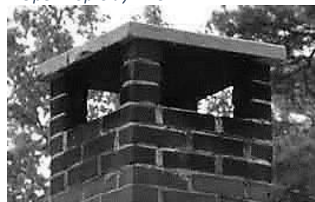
Concrete Cap Chimney Top
