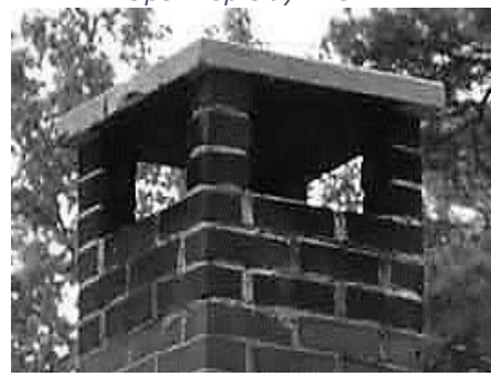
Concrete Cap Chimney Top
