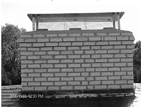
Metal Cap on Clay Liner Chimney Top
