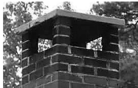
Concrete Cap Chimney Top
