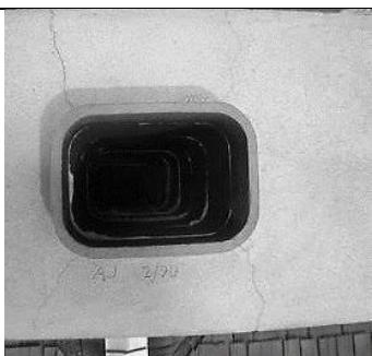
Clay Tile Liner Flue
