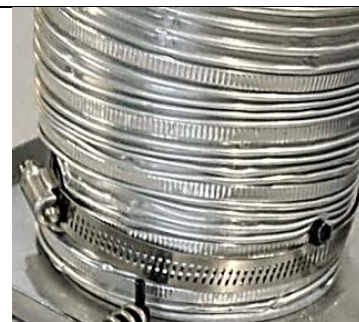
Vent Adapter Flex Connection Hose Clamp first. Secure w/ Screw above Hose Clamp
