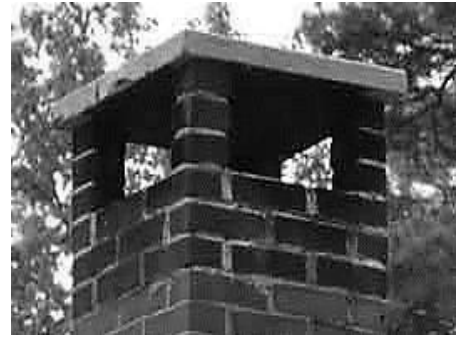
Concrete Cap Chimney Top
