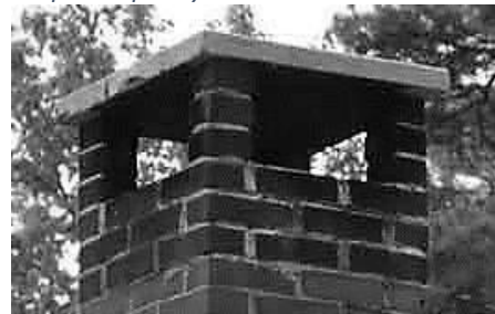
Concrete Cap Chimney Top
