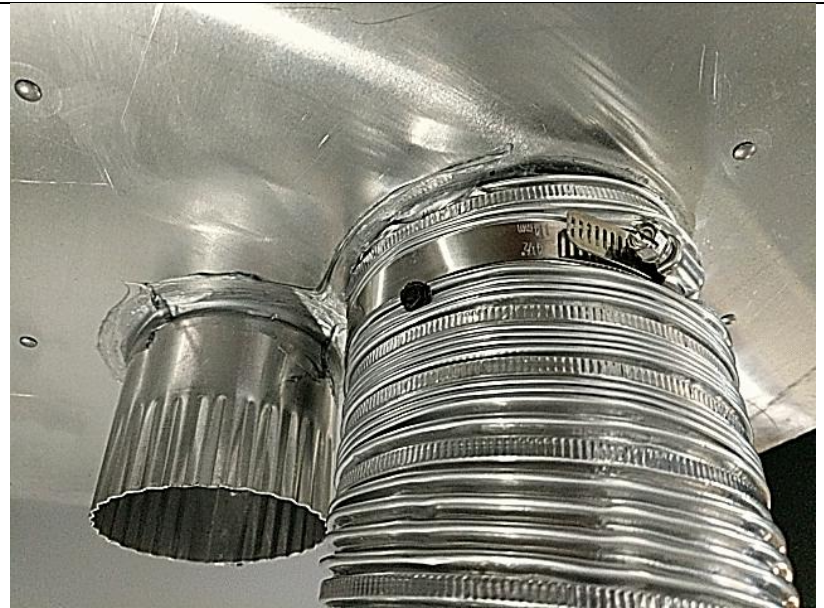
Vent Cap Flex Connection Hose Clamp first. Secure w/ Screw below Hose Clamp
