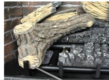
Log "G" position on front grate
